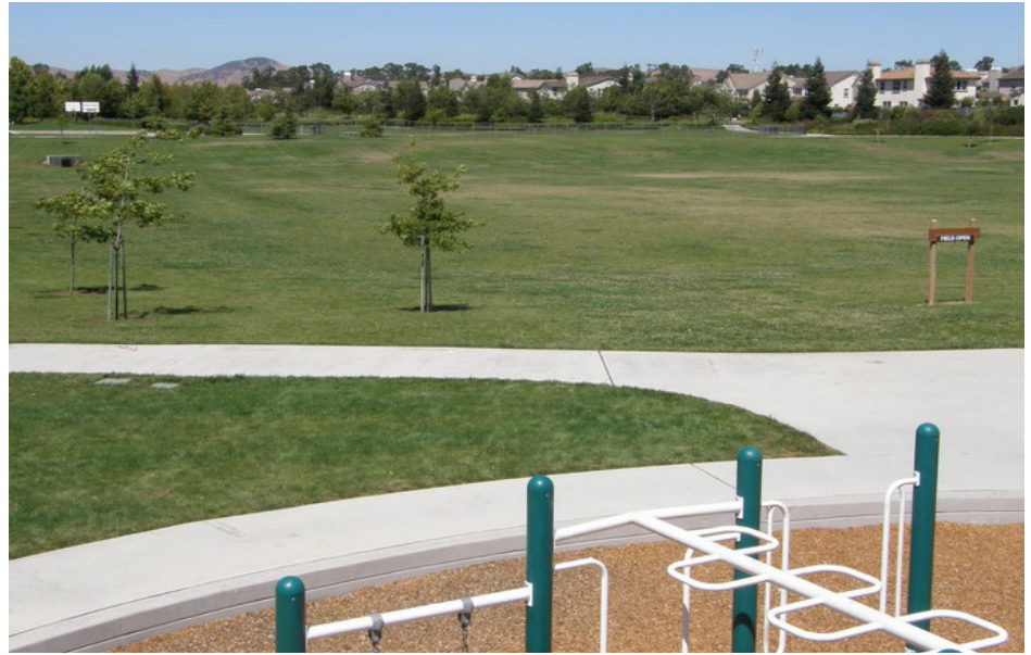
A shallow bowl can function as a playfield in summer and a detention pond in winter, allowing for the slow infiltration of stormwater. An outlet keeps the basin from flooding in large storms (Bruno Canziani Park, Livermore.)
