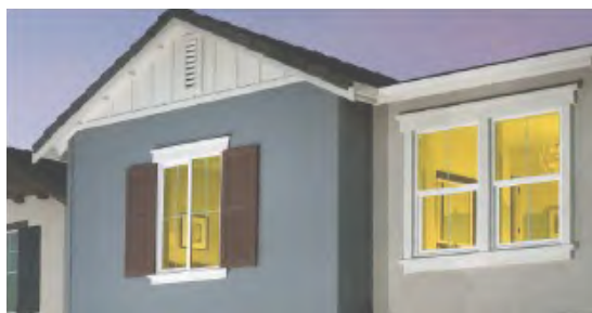
Architectural breaks make good material transition areas.
