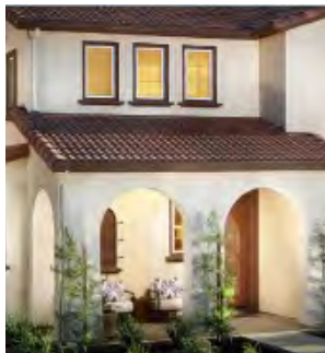
Stucco Exterior Walls
