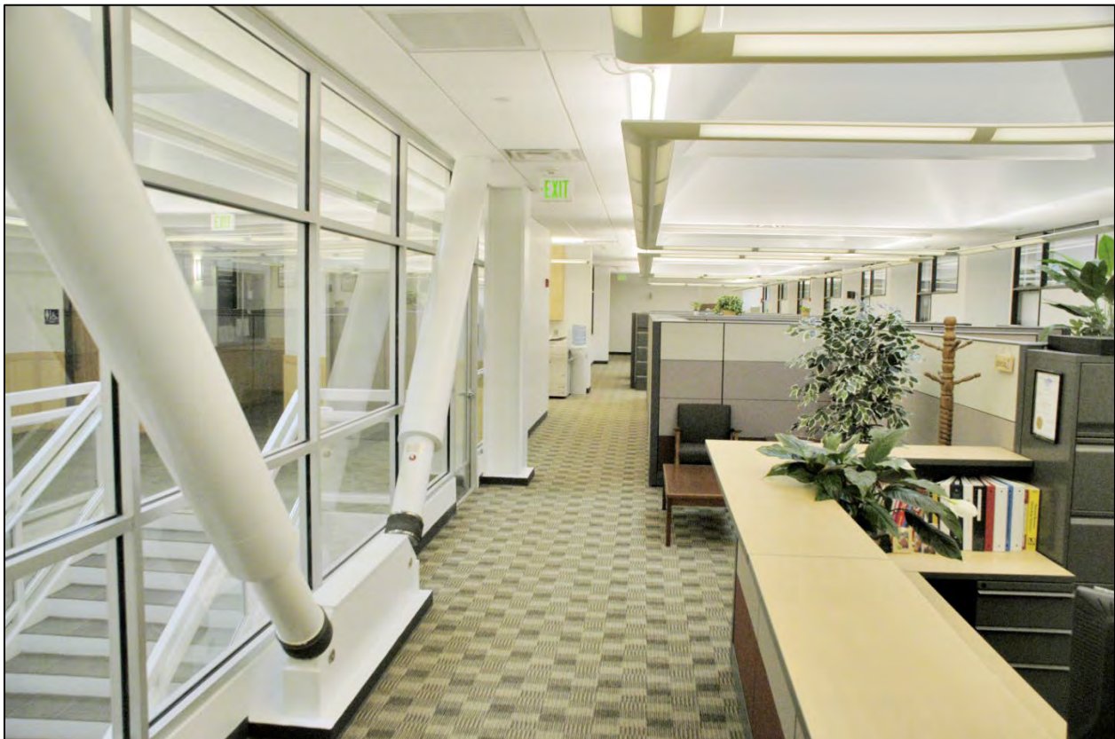
Figure 59 - Earthquake Protected Police Building with Seismic Dampers & Daylighting, Vacaville, CA
