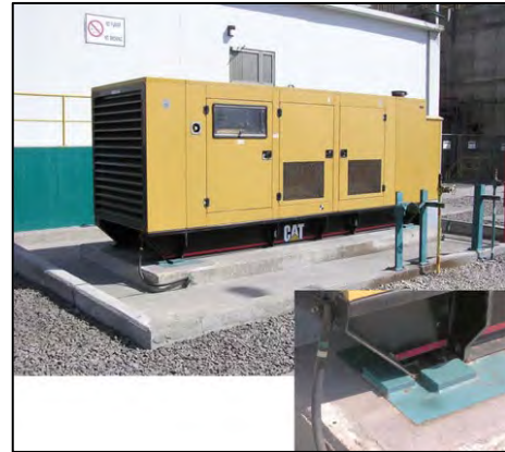
Figure 58 – Emergency Generator with Shear Lugs Added to Seismic Skid Mount
