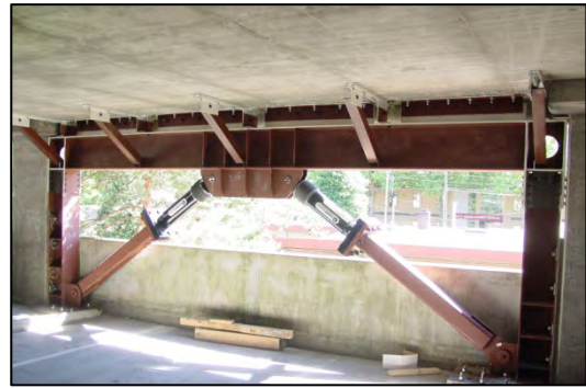
Figure 53 – Viscous Damper Retrofit, Kent WA
