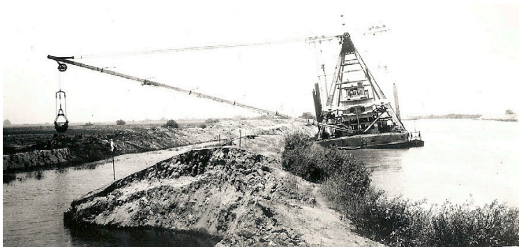
This early 1900s photograph showing early dredging work on a levee. (Covello ca. 1900, courtesy of Bank of Stockton Historical Photograph Collection)
