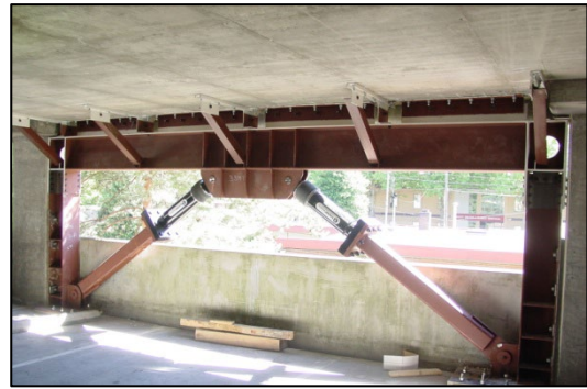
Figure 55 – Viscous Damper Retrofit, Kent WA
