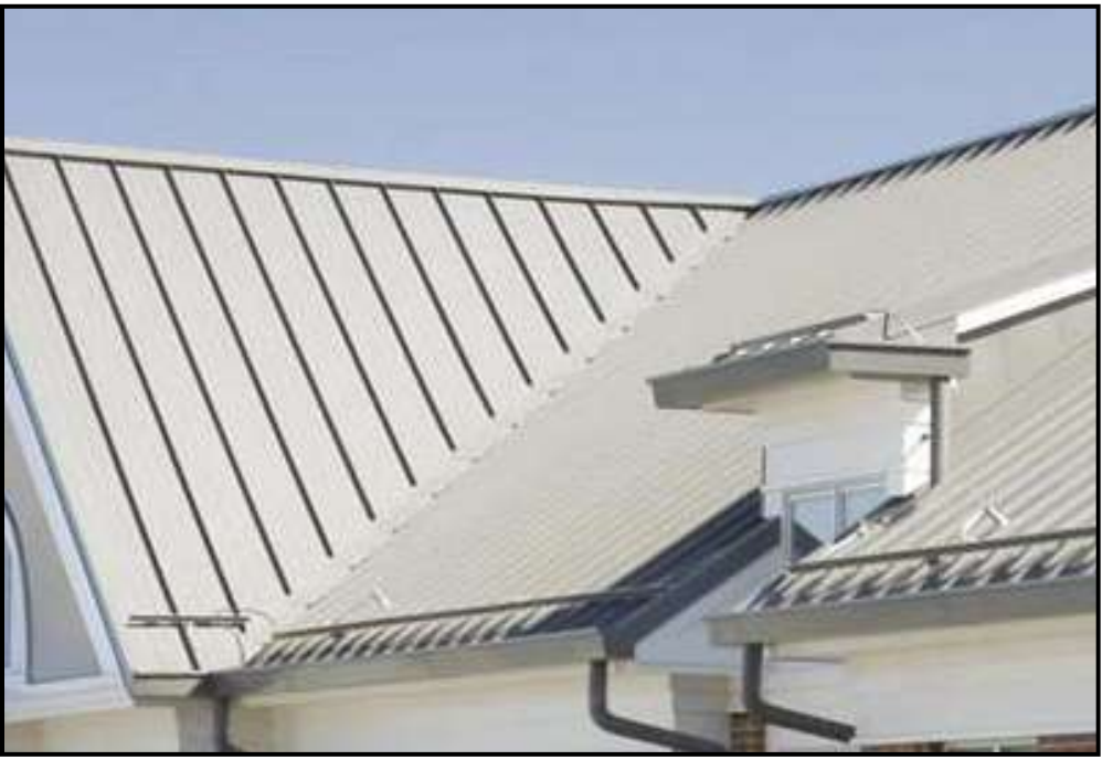
The Garland Company Standing Seam Roof
